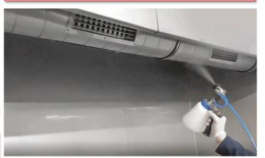
Ventilation systems: For the targeted disinfection of the air inlet you will find the nozzle for the larger throw range in the scope of delivery.
